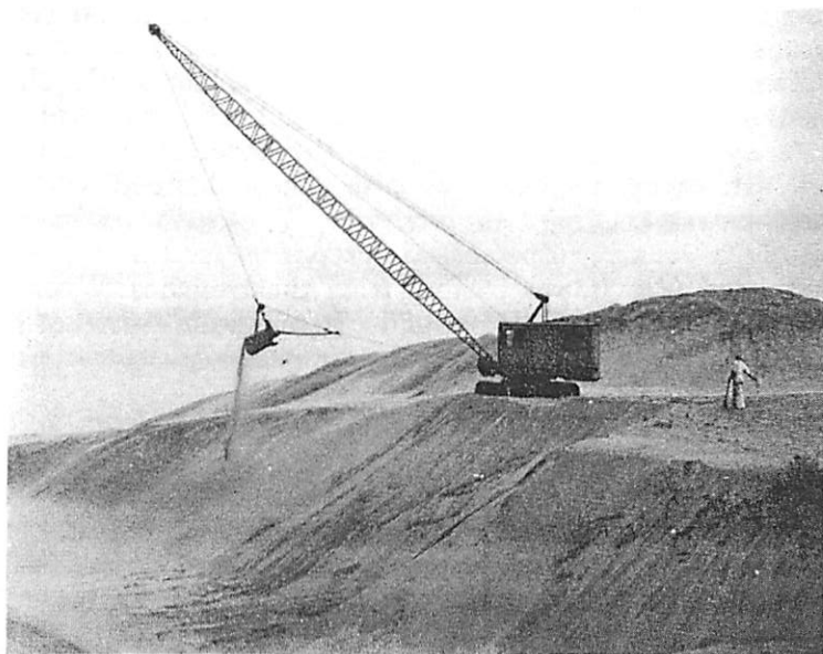
Drag line opening western end of prospecting trench removing overburden (Photo T. McNally)
