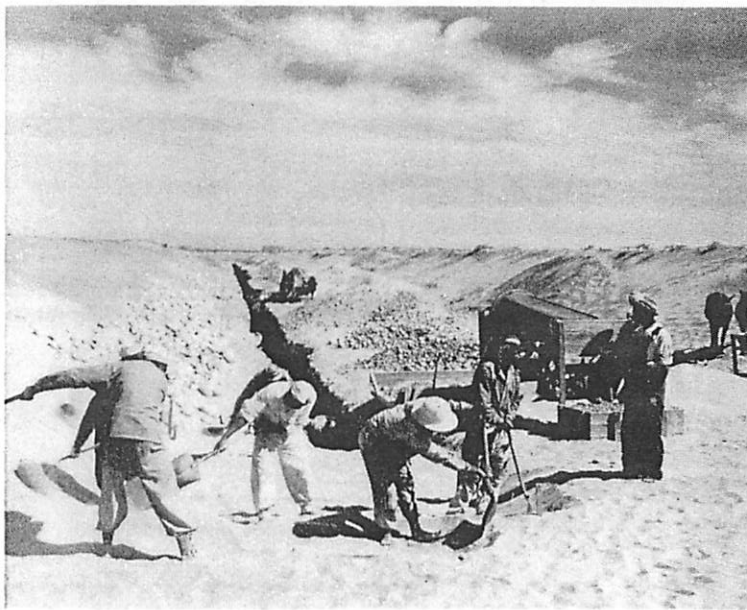
Trenching - foreground - removing soft sand to expose diamond bearing material (Photo T. McNally)
