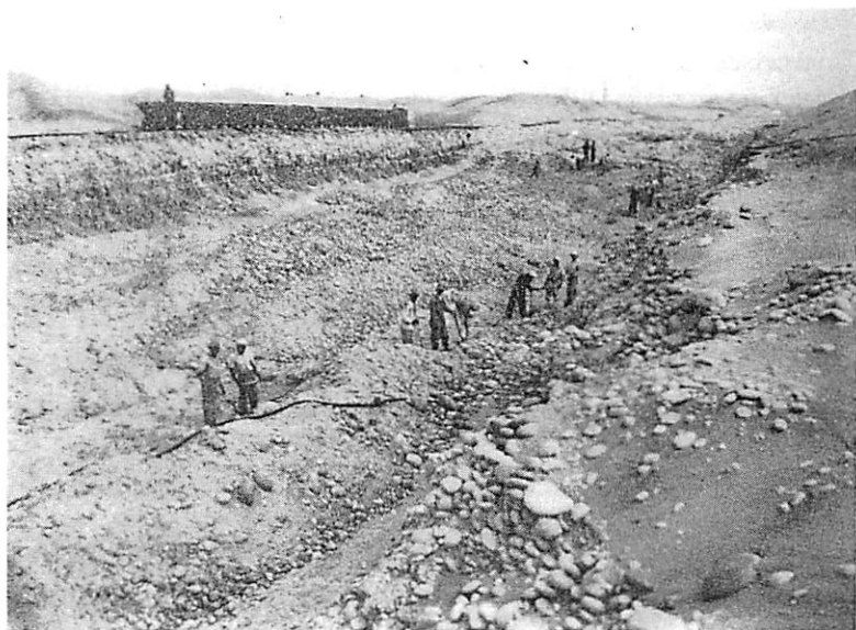
Bedrock Cleaning - note amount of physical handling of material (Photo T. McNally)
